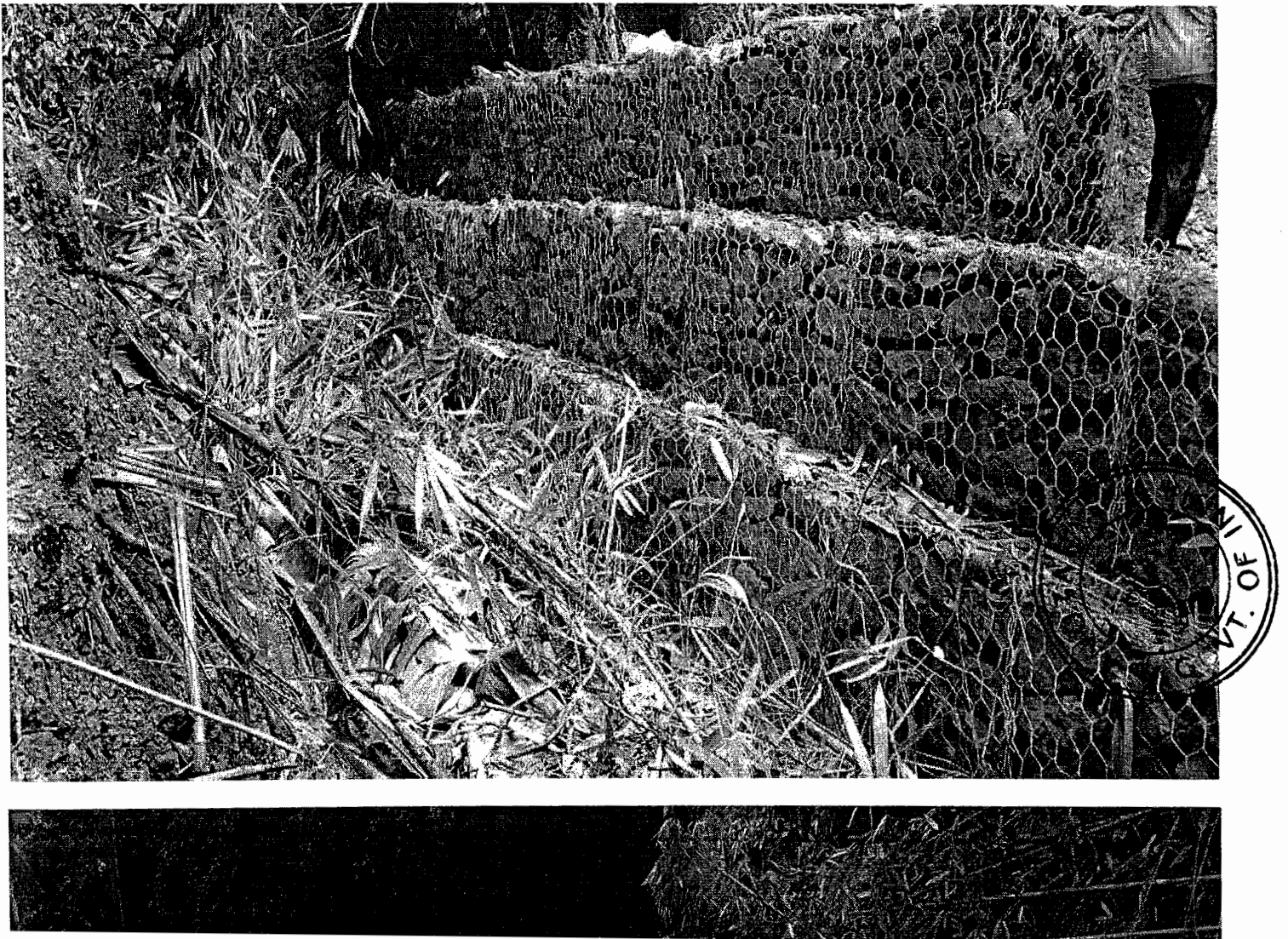
PHOTOGRAPHS OF Add. SPOIL BANK CH-256+540 TO 256+600
